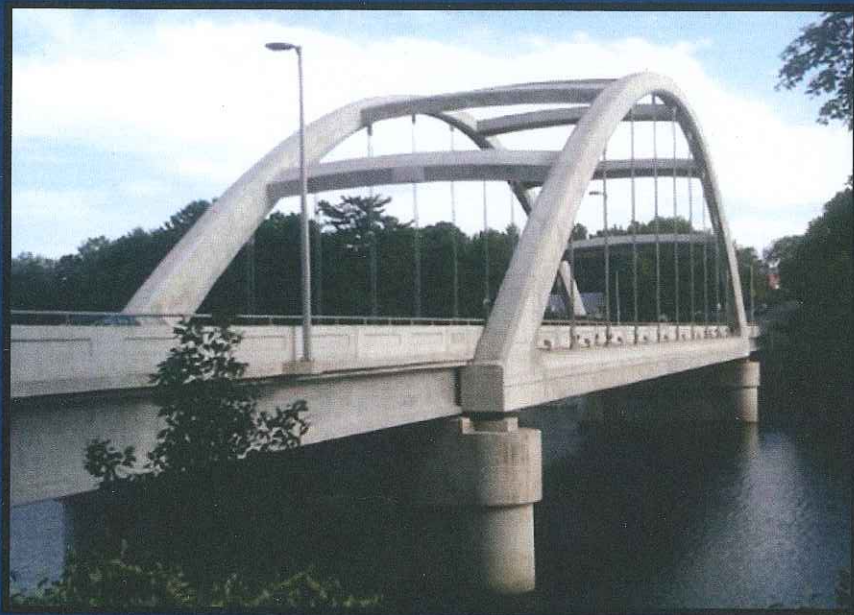
Conventional (Norridgewock Covered Bridge)
